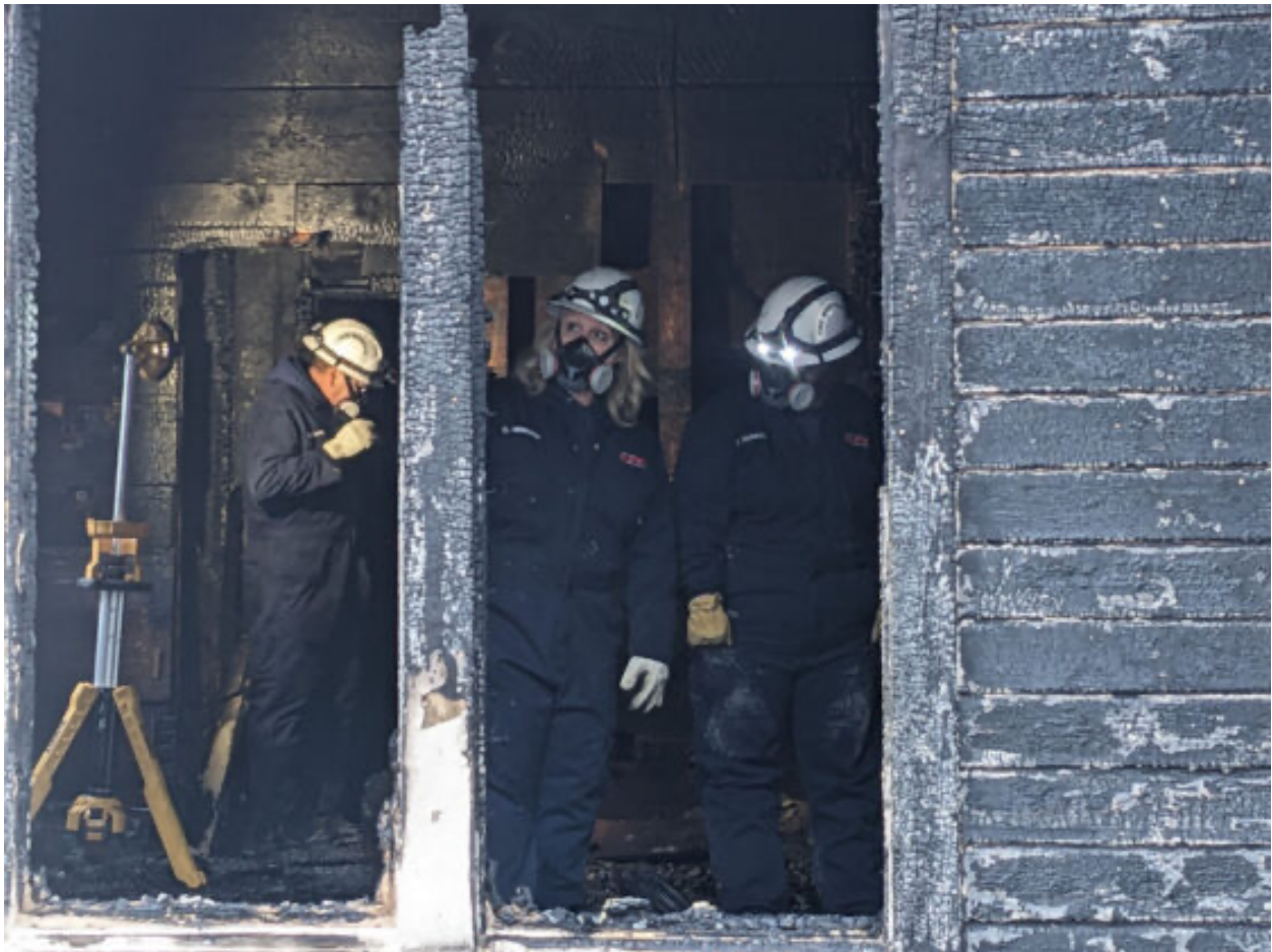
Firefighters inspect a burned-out house on Park Street on the morning of Dec. 24, 2023. Photo by Sarah Brown
